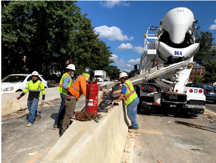
Picture No. 1: 10/05/2020 – Concrete placement for the concrete barrier (West View)
