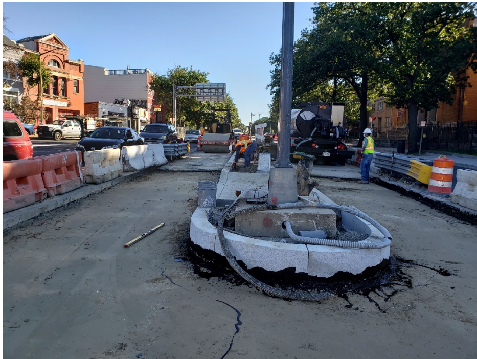
Picture No. 8 – 10/08/2020 – Placement of tack coat along NY Ave and NJ Ave intersection (East View)
